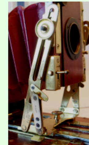
V. Cranked arm at the front and a straight arm behind, complete with locating pins in the lens panel
